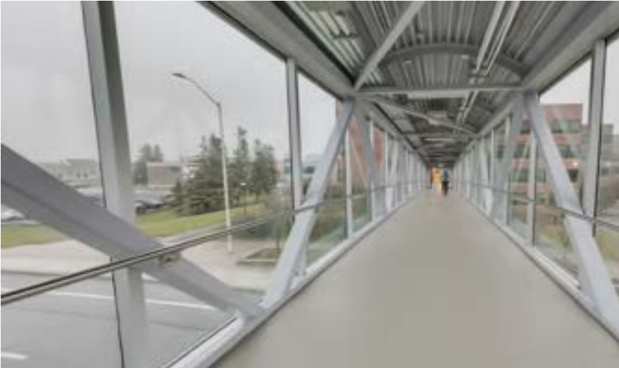
Pedestrian Bridge Between ACCE and Building B Over Woodroffe Avenue
