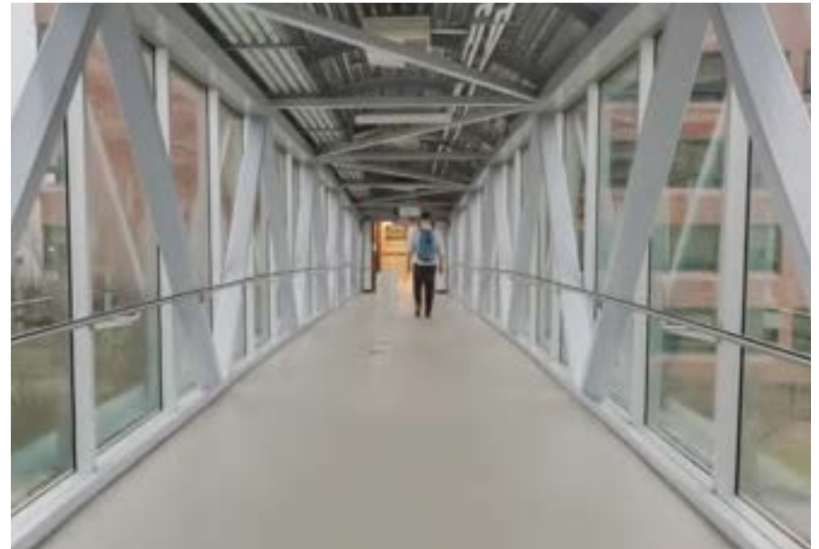
Pedestrian Bridge Between ACCE and Building B Over Woodroffe Avenue
