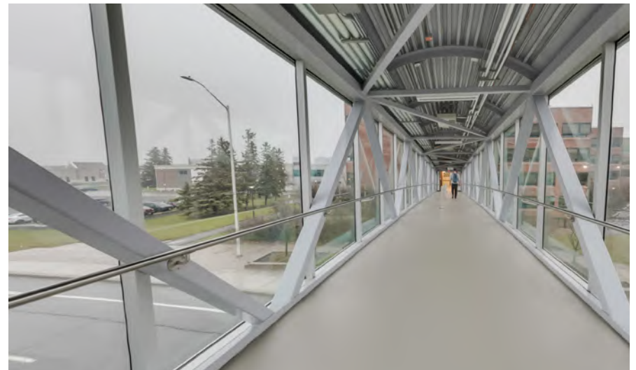
Pedestrian Bridge Between ACCE and Building B
