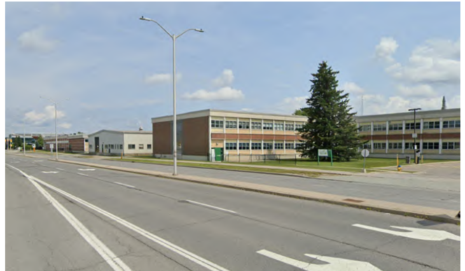
Building A from Navaho Drive
