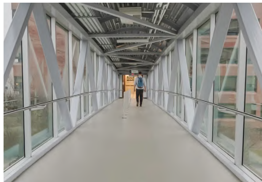
Pedestrian Bridge Between ACCE and Building B
